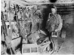
Figure 30: Photograph was taken near Loos in France on 31 January 1918 and displays rescue equipment used by the 3rd Australian Tunnelling Company during the First World War. The cages in the foreground were used to carry mice or canaries, which were used to detect the presence of poison gas. 152
